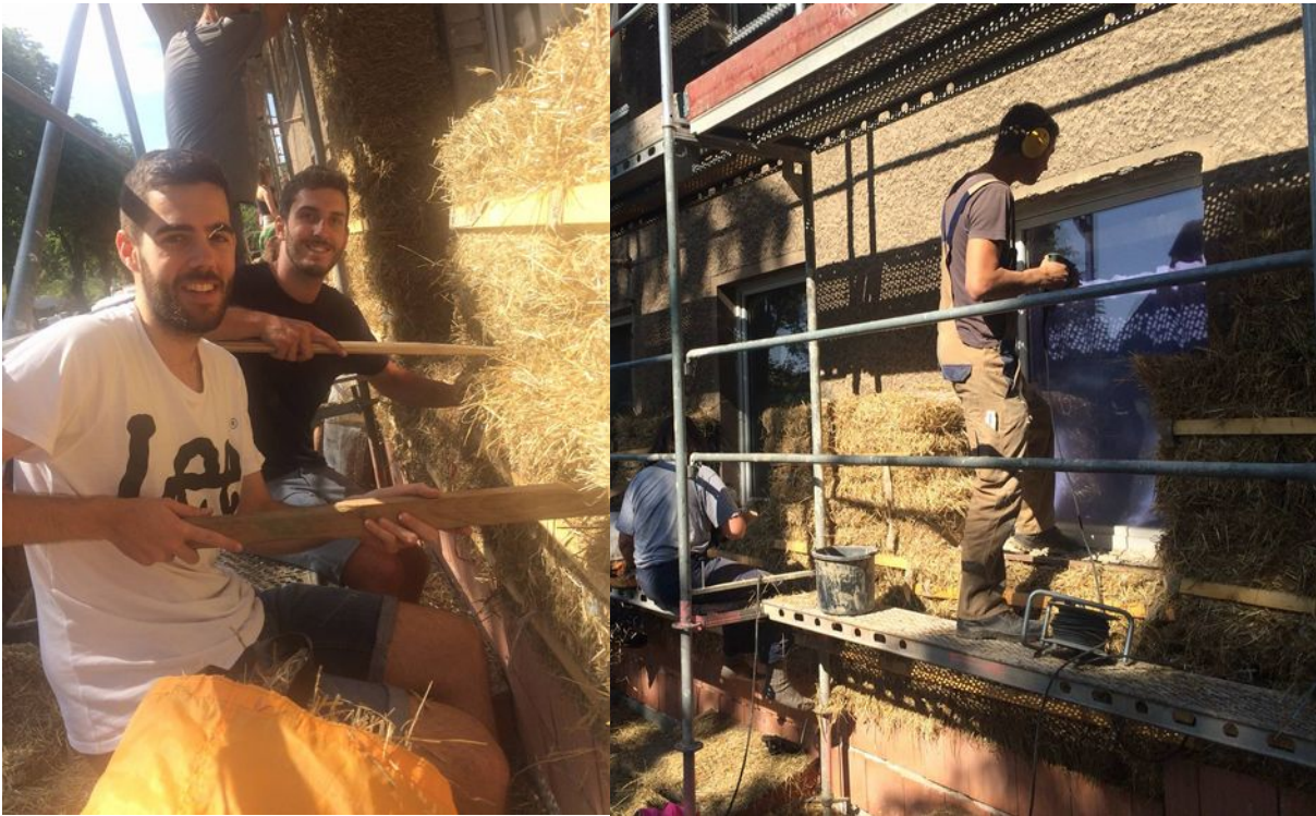
thermal insulation with straw
